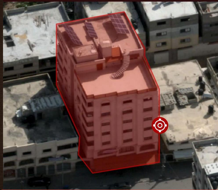
Hamas operational HQ located in a residential building - Jabalia, Gaza Strip, 09.10.23
